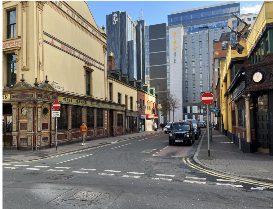
Photo: Existing Amelia Street Road Condition
