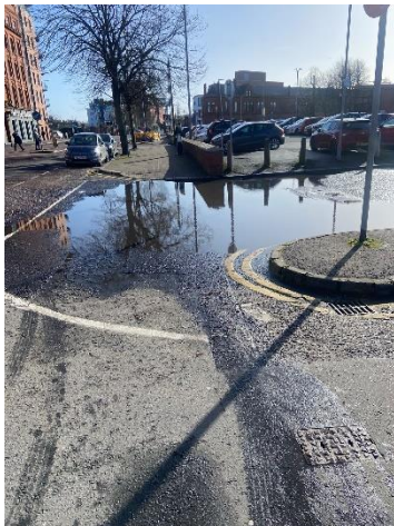
Bankmore St / Ormeau Ave junction (entrance to Charlotte St car park) flooded road surface (due to blocked drain?)
